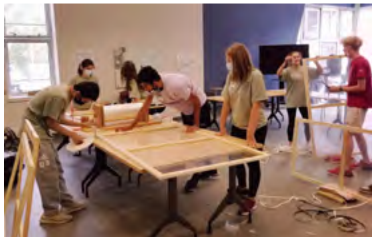
Residential students built interior storm windows in ATEC as part of a weatherization project with the Community Housing Improvement Program (CHIP).
